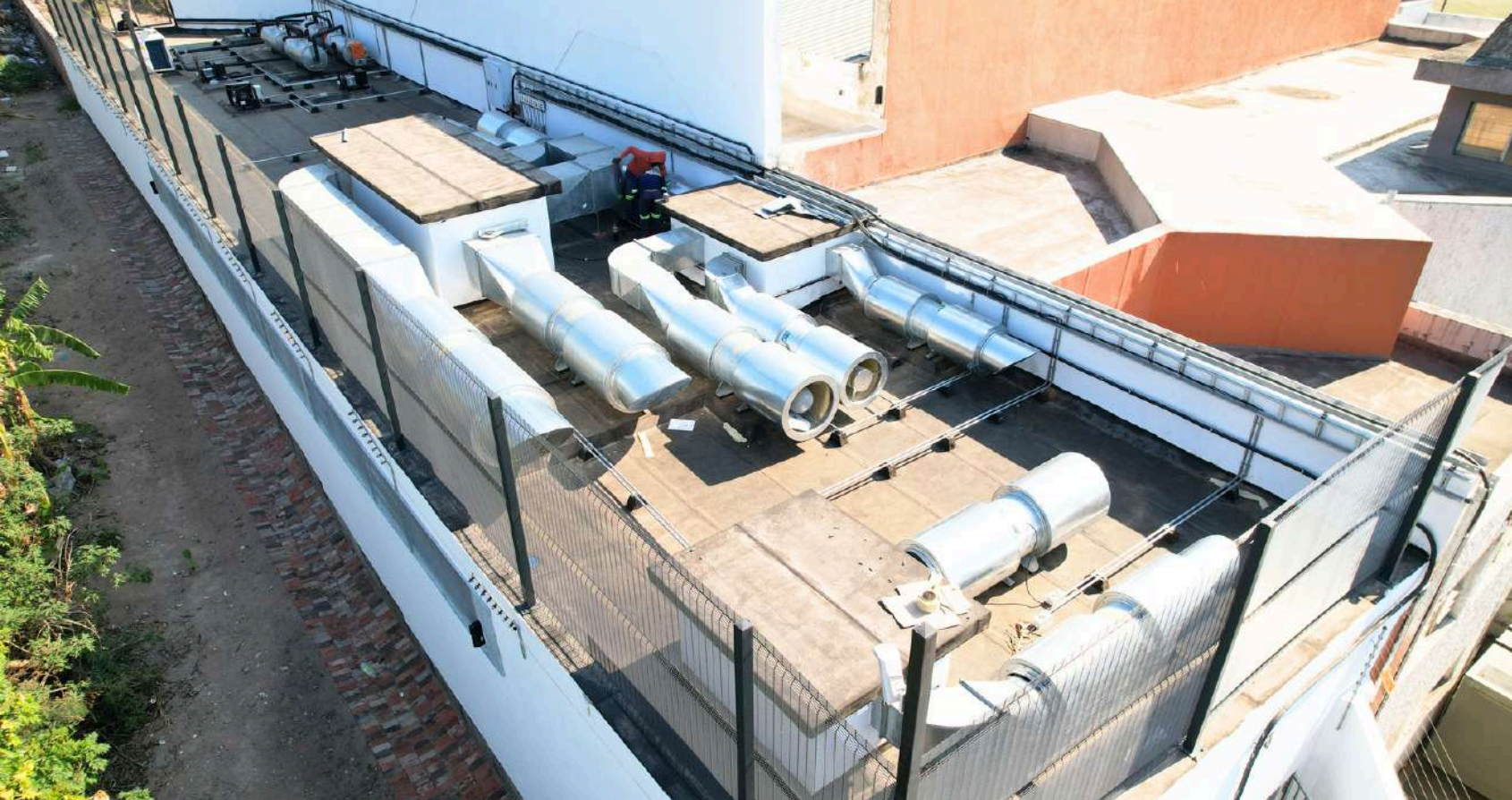
Roof Level installed with Ventilators, Makeup Air ducts, Compressors and Electrical supply to the Compressors
