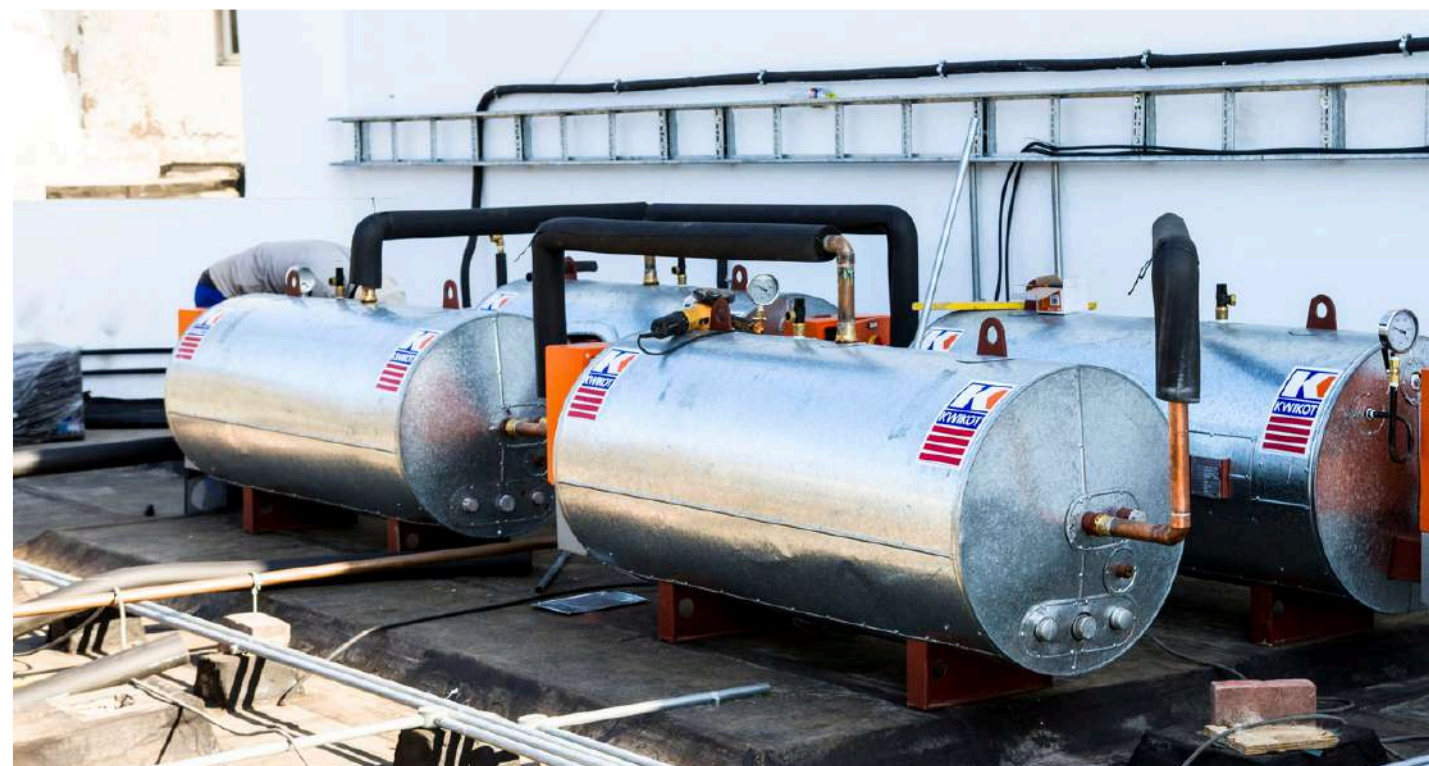
Heated Water Supply system
